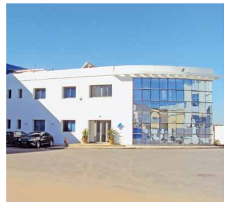
Some 35 kilometers from Tunis – Medpack, Tunisia's biggest print shop project and fully equipped with Heidelberg machines.
