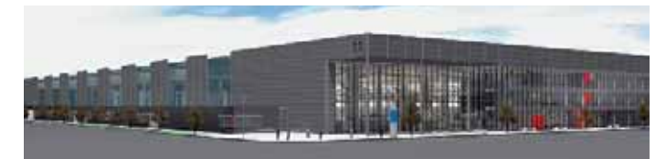
Gigantic: the future production halls for the new 6 and 7b presses, the Speedmaster XL 142 and XY 162 models, are currently under construction at the Wiesloch site.
