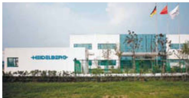
Officially in operation: The new Heidelberg plant at Qingpu near Shanghai in China.
