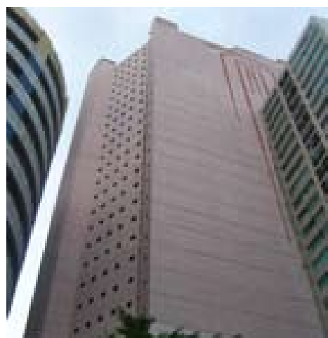
Heidelberg's Logistics Quartet Completed in April: Alongside its counterparts in Germany, the United States and Japan, the hub for replacement parts in Hong Kong ensures worldwide availability of parts.
