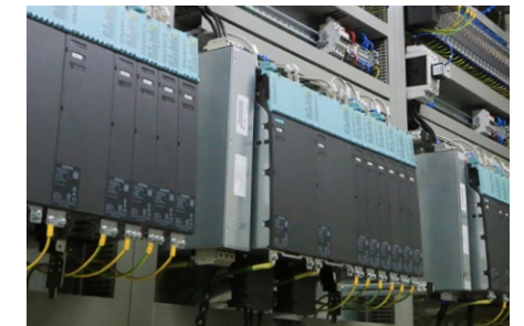
Electronic components are stored compact, easily accessible, free of dust and at a constant temperature in the e-container.
